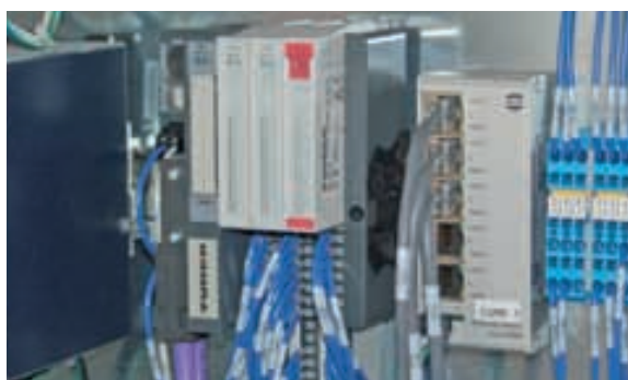
BL20 I/O systems installed within the subassembly give users control and diagnostics on the machine
