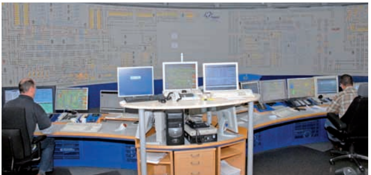
All information is collected at the control center of the automatic baggage transportation system in the airport
