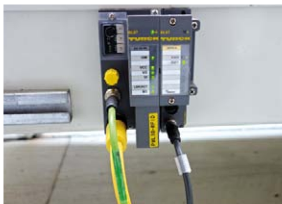
Turck's BL67 gateway transmits the data via Profinet to the PLC
