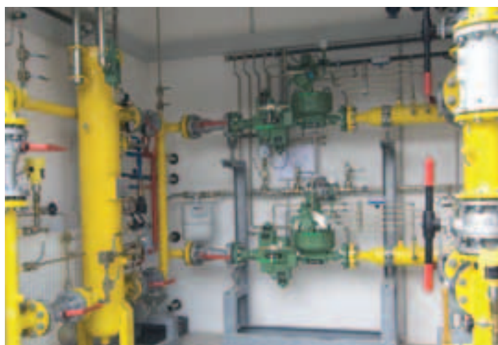
Temperatures, pressures and other measurement signals are recorded and transferred to the control room via remote service
