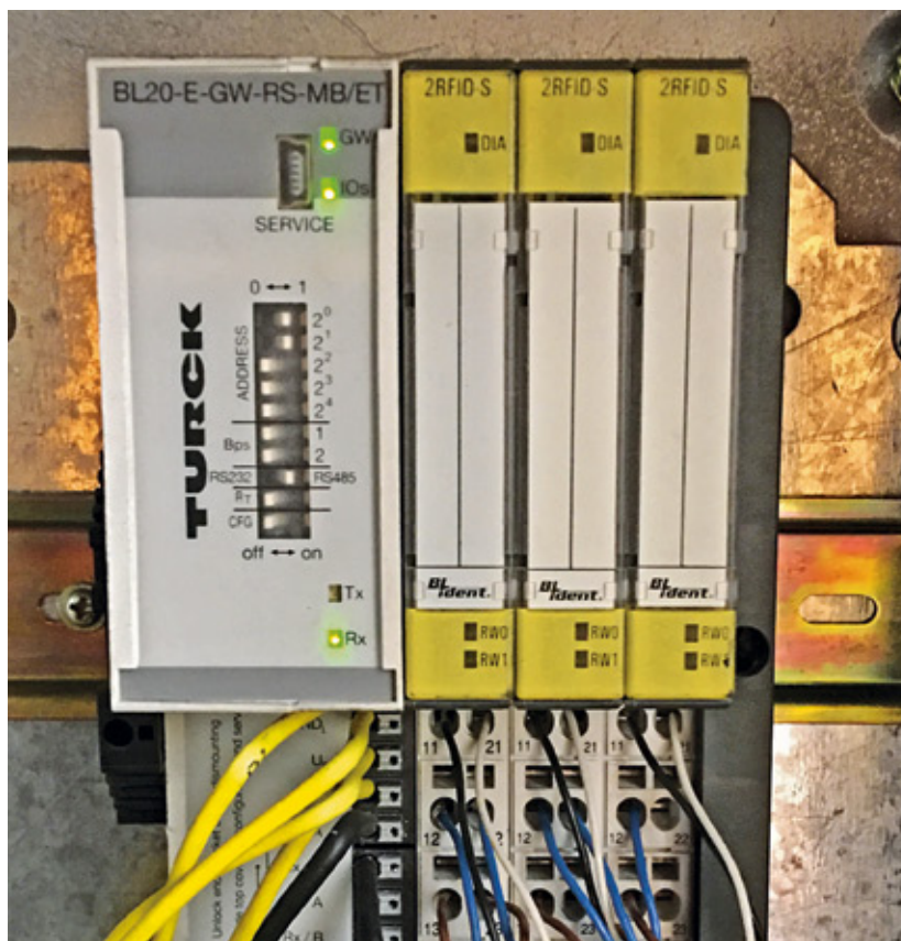
The BL20 gateway with an RS485 connection provides communication to the controller, while the RFID-S slice module enables simple connection without any programming
