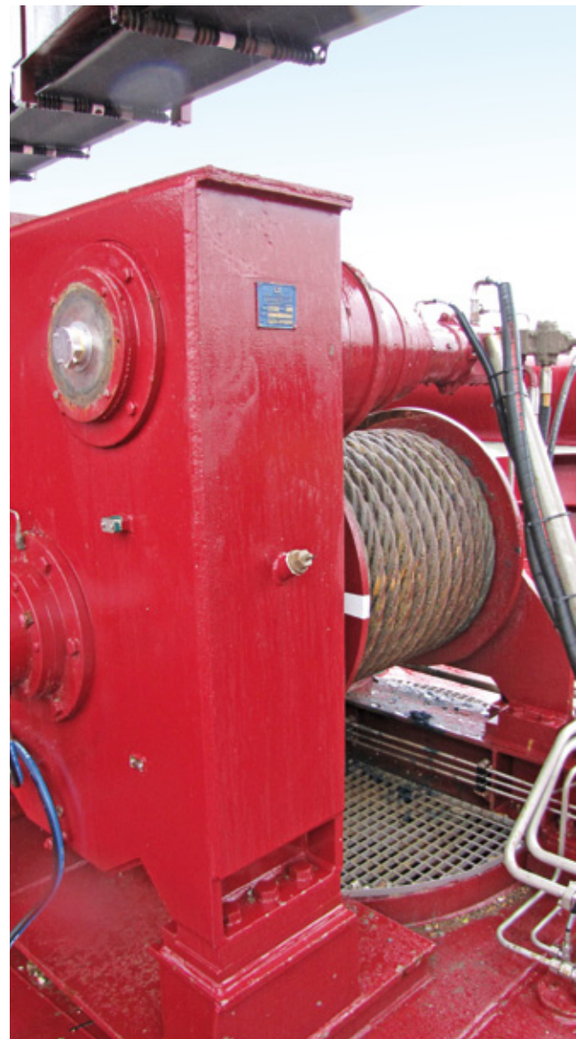
Three of these winches guide the suction pipe, at top left, an encoder detects the rotation of the shaft.
