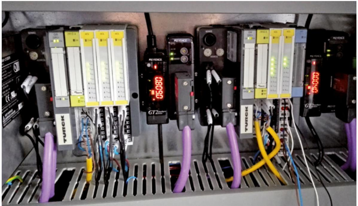
Besides hundreds of switching signals, two BL20 gateways also bring signals from RFID read/write heads and analog signals to the PLC
