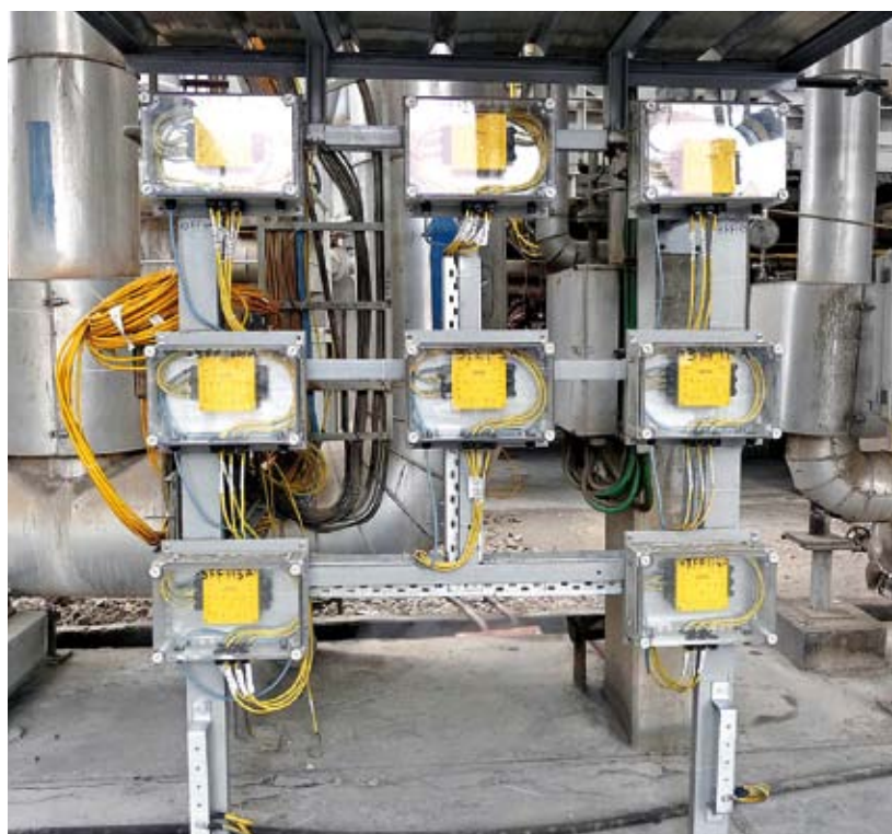
165 eight channel JBBS-49SC-T815 junction boxes from Turck guarantee a safe connection between the field devices and the DPC-systems
