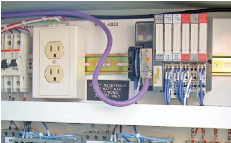
IP20-rated distributed I/O systems collect all of the signals from a local area
