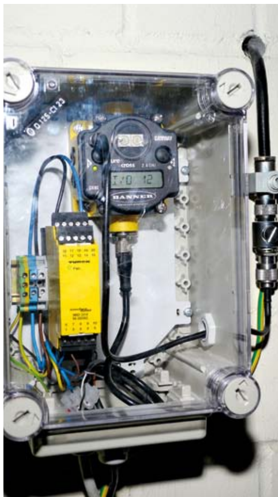
The DX80 gateway processes the radio signals and forwards them to the control room onsite and to the superior controls via Modbus RTU
