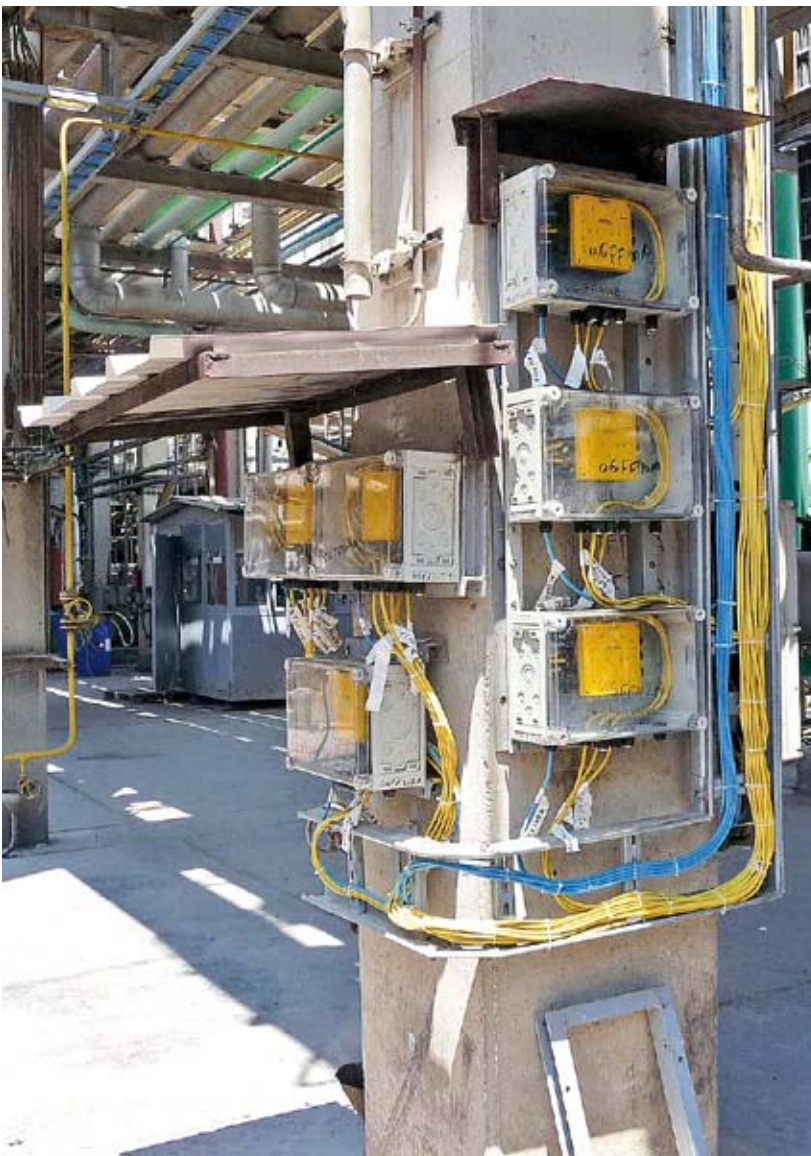
Because of the special ambient conditions in the ammonia facility, Turck placed the IP67-fieldbus components into additional protective housings
