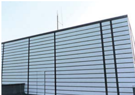
The antenna on the roof of the filter hall receives the signals of all 55 connected wells
