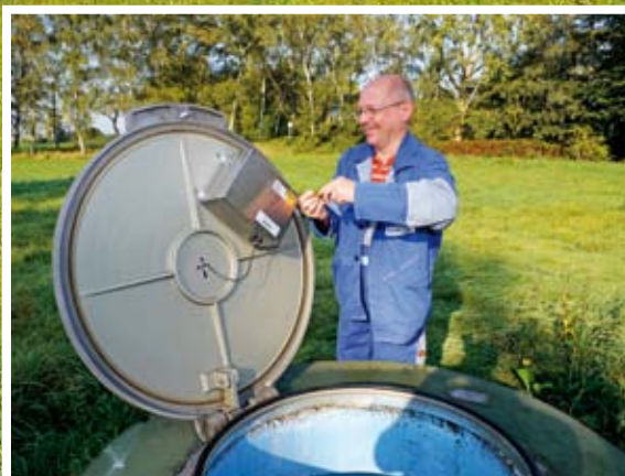
Turck supplies prefabricated systems in a stainless steel box, that has to be mounted to the well covers by RWW electrician Klaus Bitter
