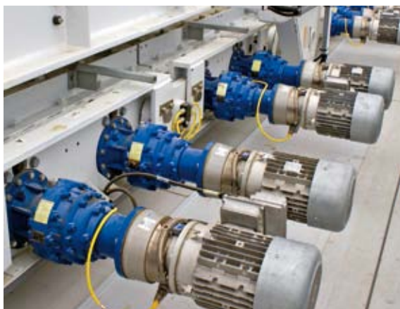
Custom-molded Turck motor cables for VFD-controlled motors
